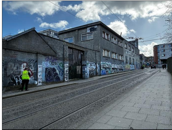
Plate 1 Photo of site from Steeven's Lane looking south
