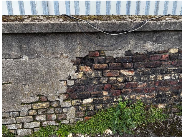
Plate 9 Close-up of the eastern boundary wall
