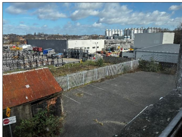
Plate 3 Shed to be demolished; yard areas will serve as the construction-phase compound and accommodate the transformer bund.
