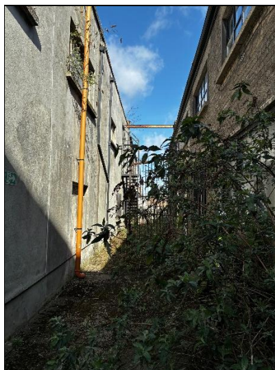
Plate 7 Walkway between the two buildings, former office on left and former factory on right
