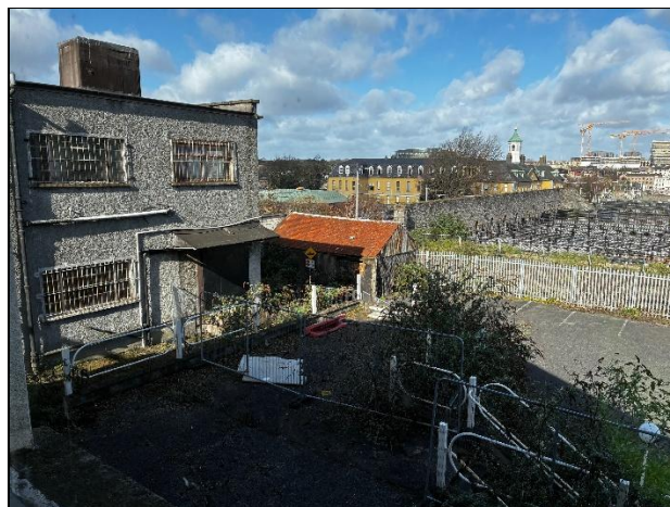
Plate 8 View of (proposed construction yard and transformer bund location) site from the upper window of the former factory building.
