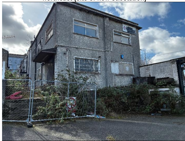
Plate 5 The former factory three storey building to be demolished
