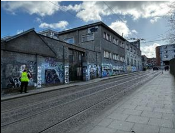
The exterior of proposed site looking southwards from Steeven's Lane
