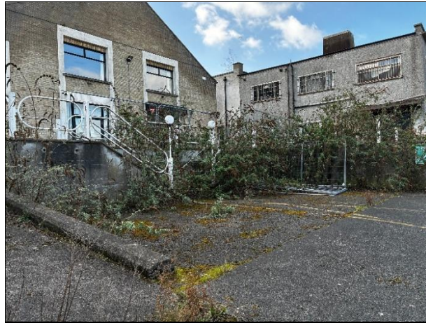
Plate 4 The two larger buildings to be demolished former office on left and former factory on right facing northeast (site of new substation)
